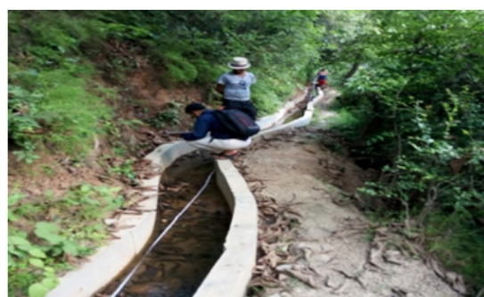
Irrigation Pond constructed (Gulmi)
